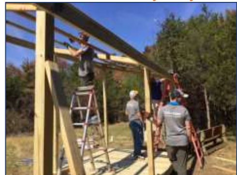
HCA Volunteers build an accessible archery deck at camp.
